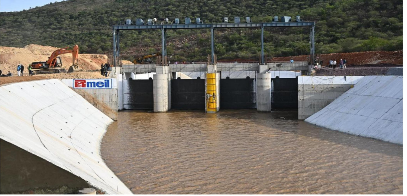
A view of the feeder canal of the Poola Subbaiah Veligonda irrigation project ahead of its inauguration in Markapuram district.
